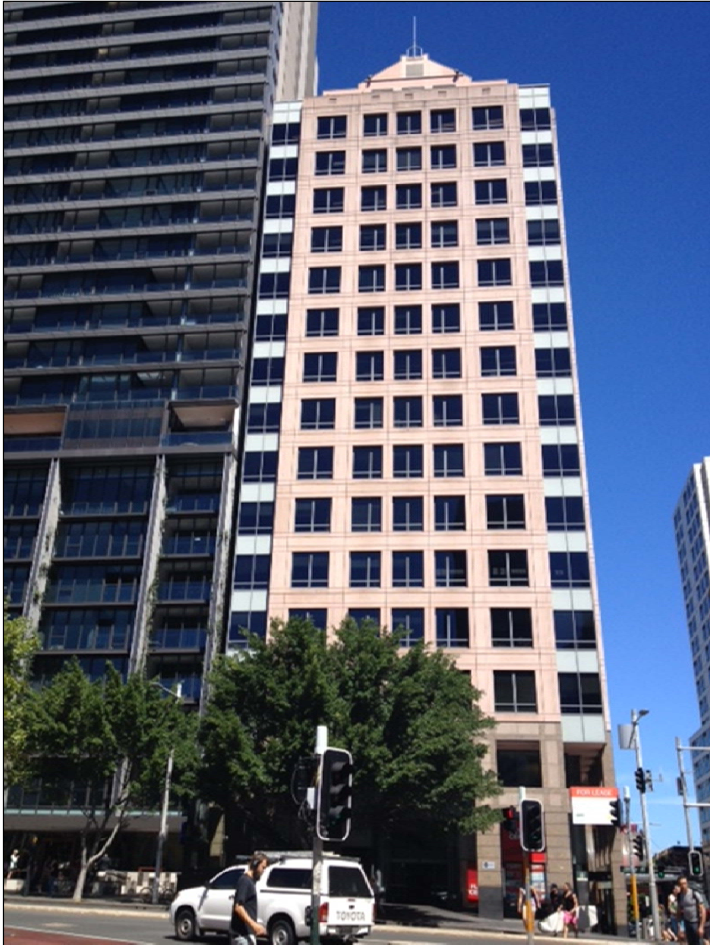
Figure 2: The existing 16-storey commercial building on site, as viewed from Liverpool Street.
